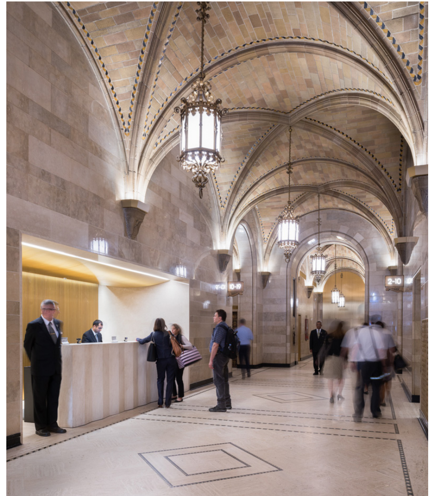
Cove lighting at the springing of each vault accentuates the repetitive rhythm and curvature of the lobby ceiling.
