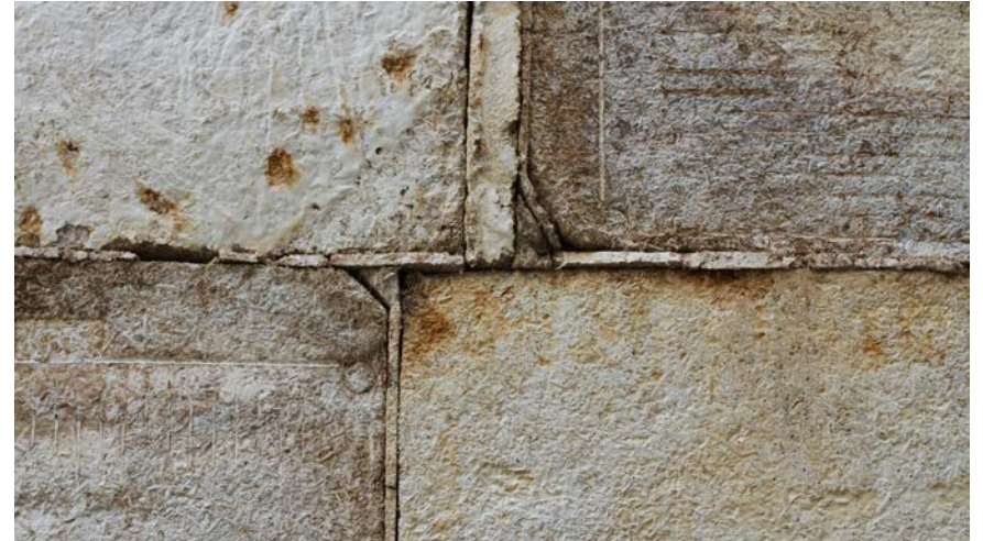
Top: Detail of assembled mycelium panels on completed installation, July 2012.
