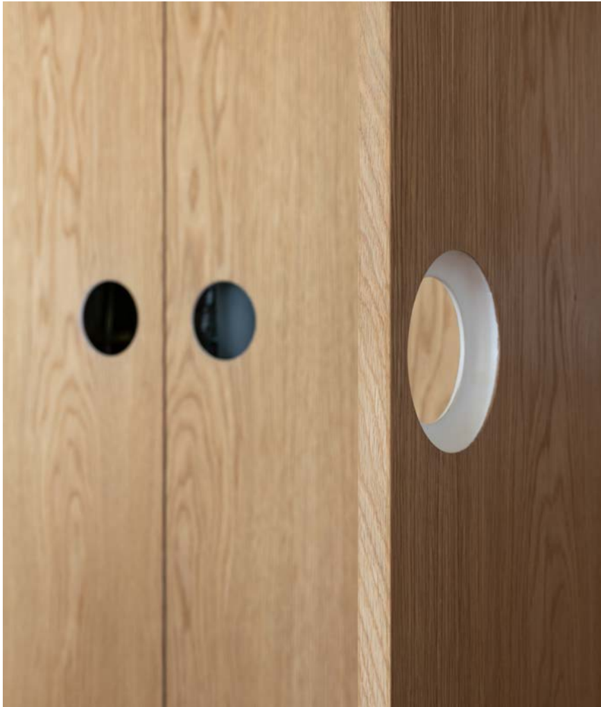
Above: A white oak millwork panel provides an insertion point for a doorknob so the adjacent stairwell door can dock flat when fully open.
