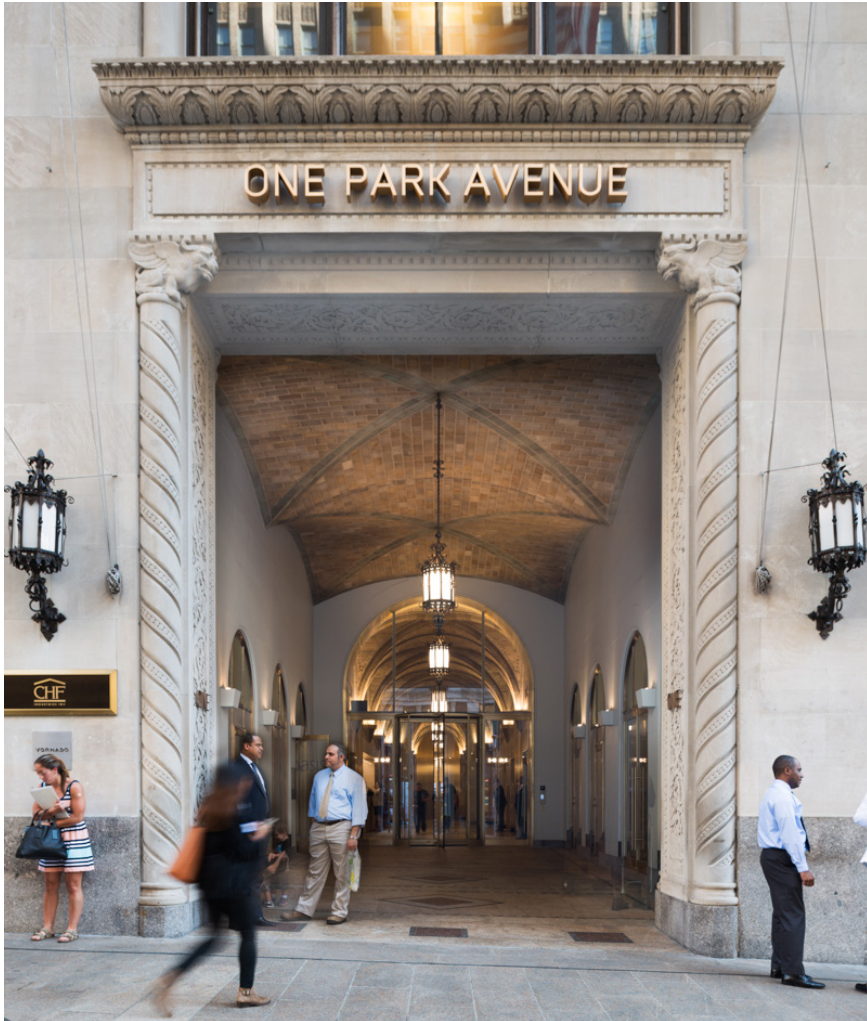
A new glass entry with a revolving door and updated signage provide a contemporary counterpoint to historic details throughout.
